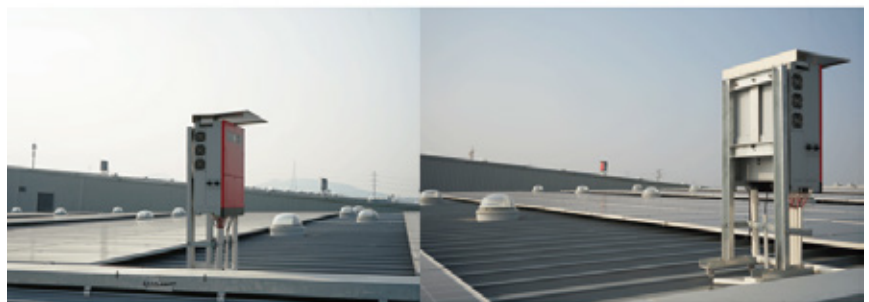
Figure 2. Inverters Mounting on Support Brackets
