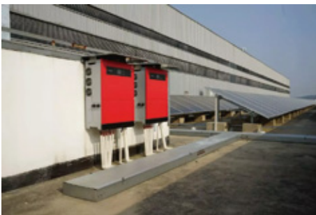
Figure 1. Inverters Mounting on Parapet Wall
